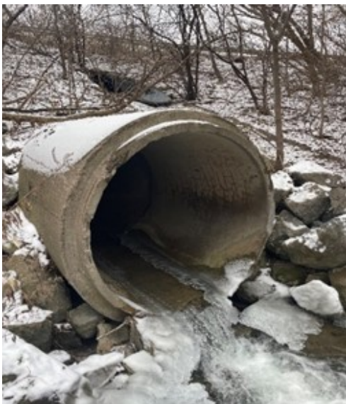
A well maintained, reinforced concrete pipe. Inspected: 1/5/22
