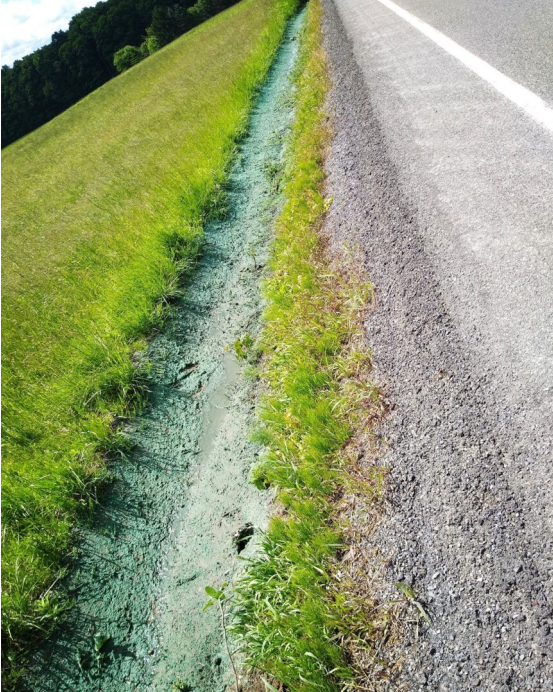
Hydroseeded Road Ditch
